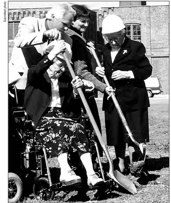
Providence Sister Mary Hickey (seated in wheelchair), assisted by Rick J. Wilson, and Providence Sister Francis Pierre Pagels (at right), assisted by Paulette Bentley, break ground for the congregation's new health-care facility for ill and infirm sisters on Oct. 7 at Saint Mary-of-the-Woods. Wilson is the construction manager for the project and Bentley is one of the project architects.
