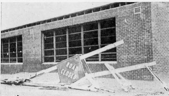
ROAD CLOSED, SCHOOL OPEN—In order to construct the four-room addition at St. Mary-of-the-Knobs school at Flays Knobs, Ind., Martin Road had to be revolved. The corner of the new addition to the 16-room ground school reaches the edge of the original road. The construction is expected to be completed by the beginning of the school year, Wednesday, Sept. 4. Two new teachers are being added at St. Mary's, staffed by the Sisters of St. Benedict and lay teachers. (Photo by Rachel Eberle)
