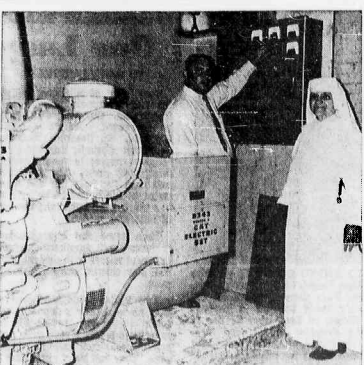
THAT $25,000 SMILE —Sister M. Vincenza, O.S.B., administrator, and Carl Hancock, chief engineer, of St. Francis Hospital, Beech Grove, proudly display a new standby electric generator which will permit normal hospital operations during power failure from regular sources. The six-cylinder diesel engine is manufactured by the Caterpillar Company. Price, $25,000. The installation, required of modern hospitals, was completed recently. (Staff photo)
